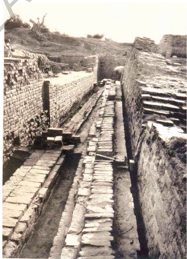
Fig. 20.8: Drainage system in a street in Mohenjodaro
