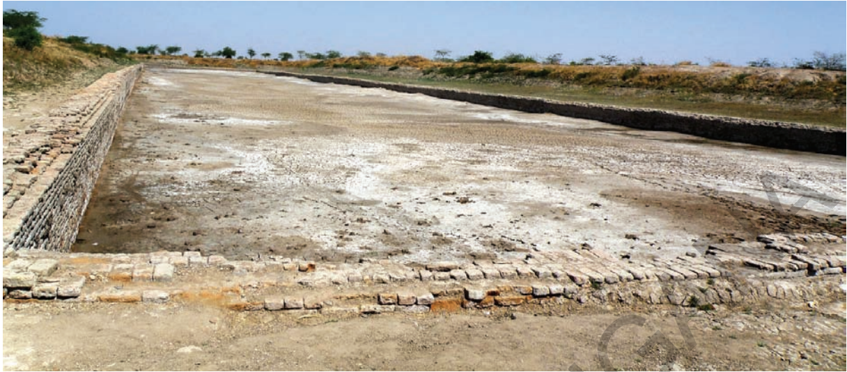
Fig. 20.5: Dockyard of Lothal - Imagine, the size of the boat that can fit here. (Dimensions 37m east-west, 22m north-south)
